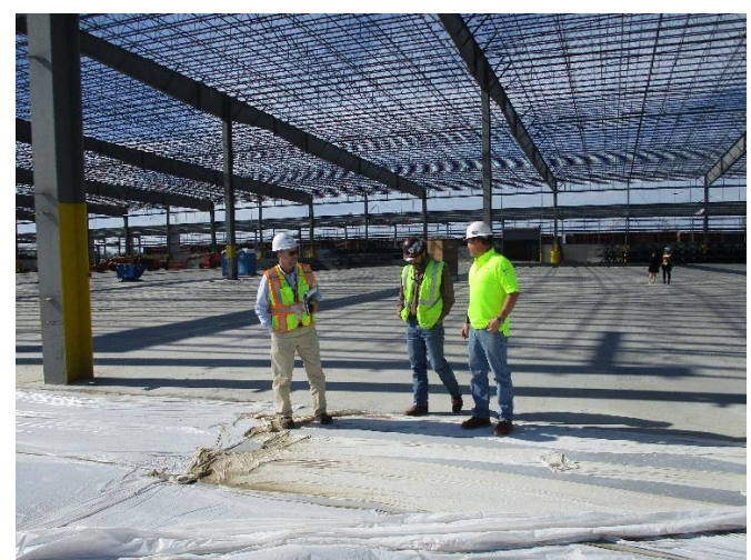
Looking Through WHSE Phase I from Expansion Slab
