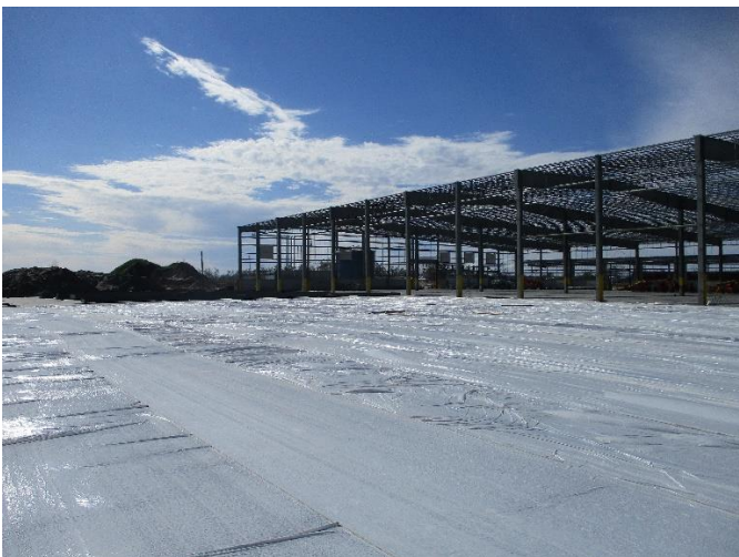
WHSE Exp. Bar Jsts. and Steel Girts Stored In Phase I
