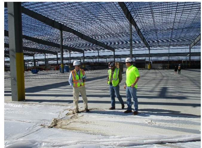
Earthwork Excavat. & Moving West Side of Site Ext.
