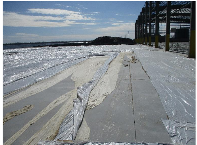
WHSE Exp. Slab Looking West (Plastic Cover for Curing)
