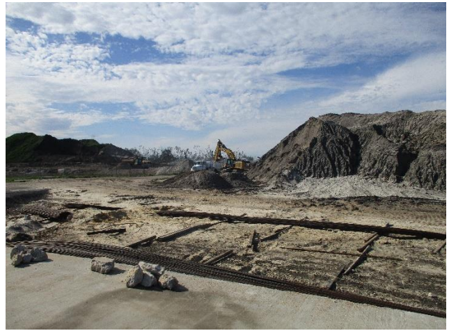
Earthwork Excavat. West Side and Stored Rebar
