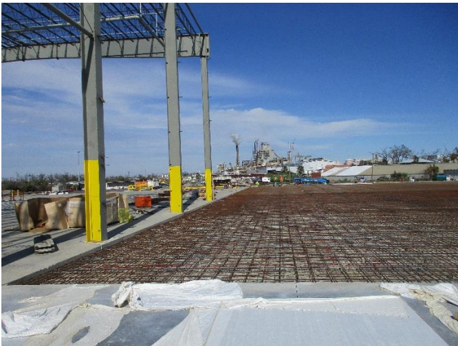
Steel Rebar Placed for East Slab Looking East
