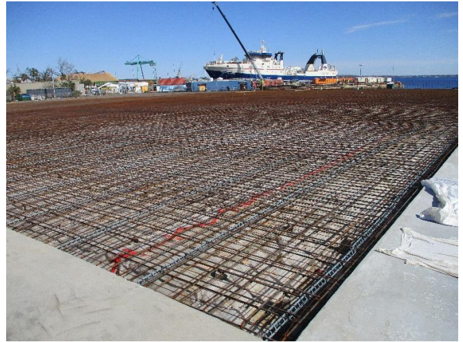
Steel Rebar Placed for East Slab Pour For This Week
