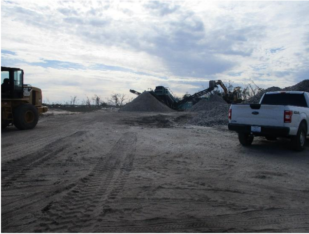
Crushing Demo Concrete for Paving Base and Fill
