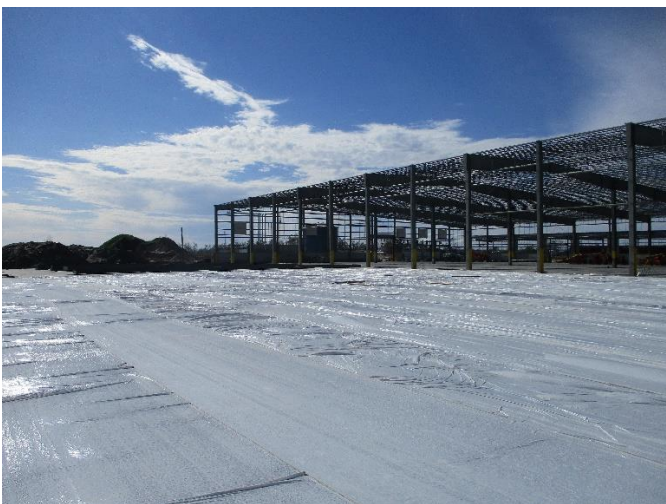
WHSE Exp. Slab Looking NW, Phase I to Right
