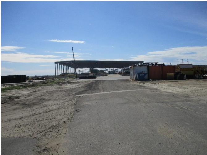
Phase I Warehouse (WHSE) Frame View West From Entry
