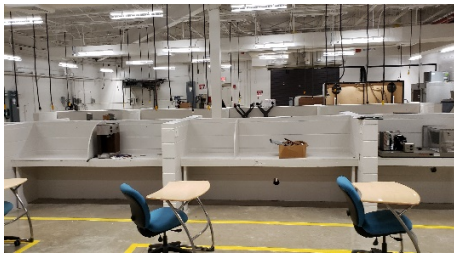
Workshop and class area, new HVAC and electric- lighting, drop cords, new panels and distribution to work stations
