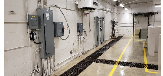
Workshop and class area, new HVAC and electric- lighting, drop cords, new panels and distribution to work stations
