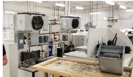
Workshop and class area, new HVAC and electric- lighting, drop cords, new panels and distribution to work stations
