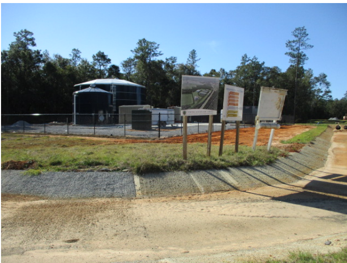
Potable And Fire Protection Water Tanks
