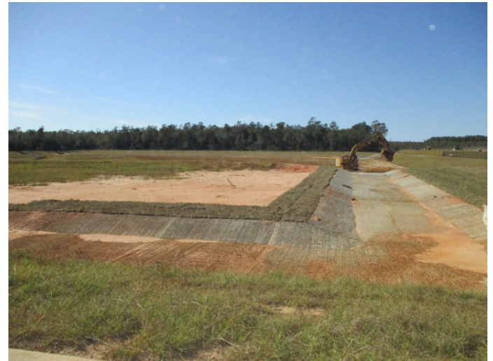
Concrete Storm Water Drainage
