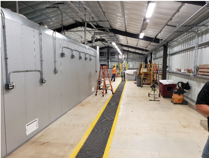
Interior lab rooms and tanks. Electrical being installed.
