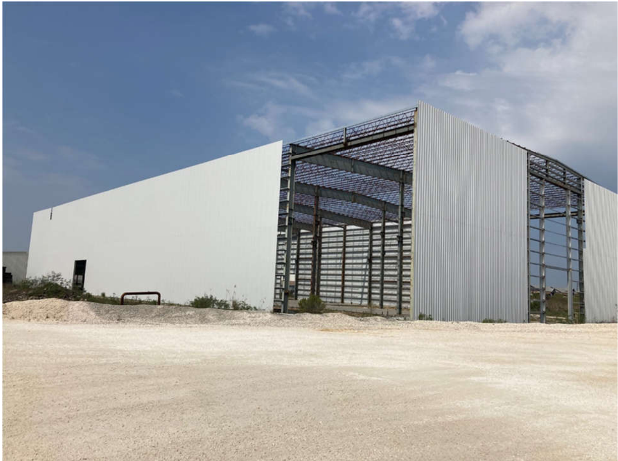
Existing condition - Warehouse 10 at Port of Pensacola
