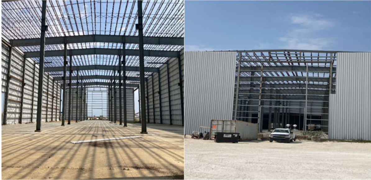
Existing condition - Warehouse 10 at Port of Pensacola
