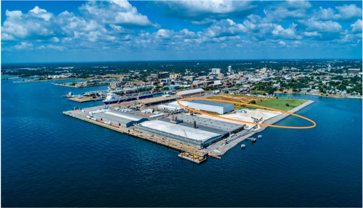
Drone photo of Port of Pensacola pre hurricane Sally. Warehouse and approximate project area circled.
