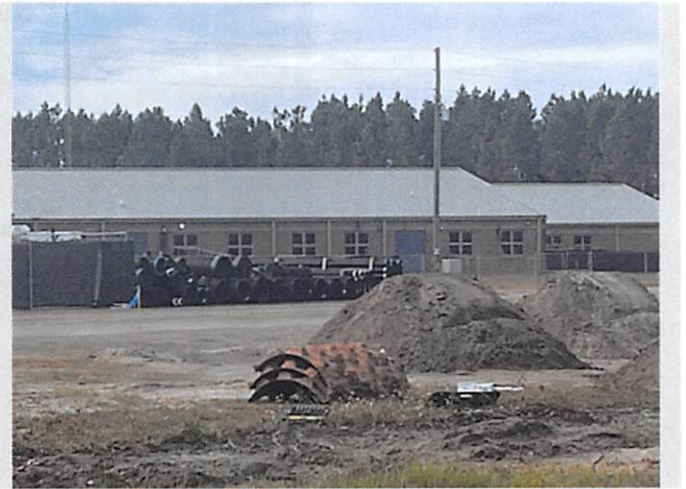
Description Storm/Sanitary/Water Pipe Delivery - On-Going
