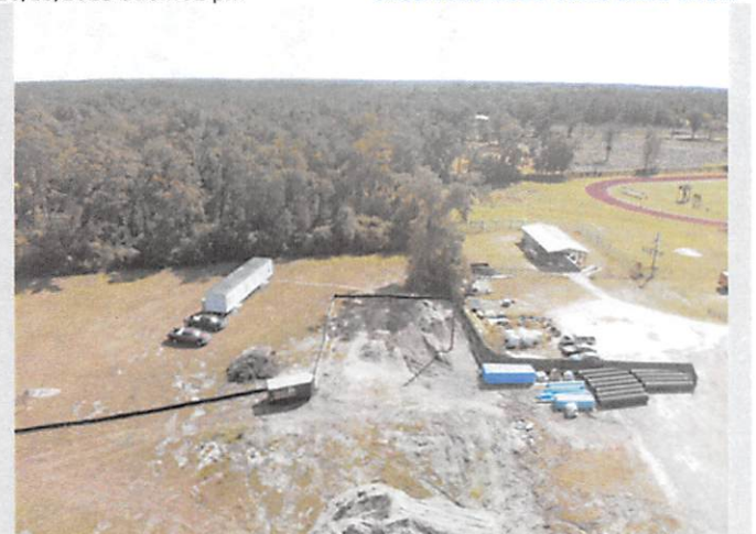
Description Aerial Photo - Job Site Overview
