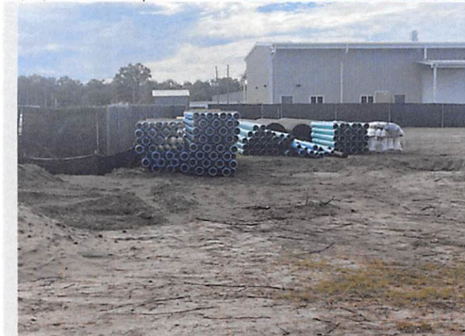
Description Storm/Sanitary/Water Pipe Delivery - On-Going
