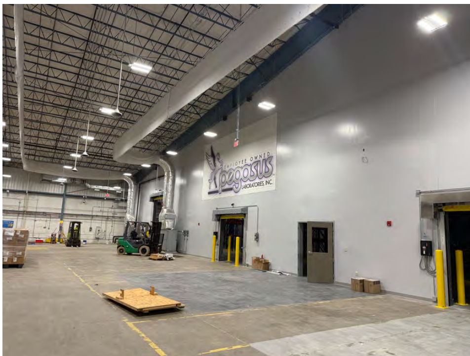
Upgrading HVAC for Climate Control (requirement of Pharmaceuticals after production)
