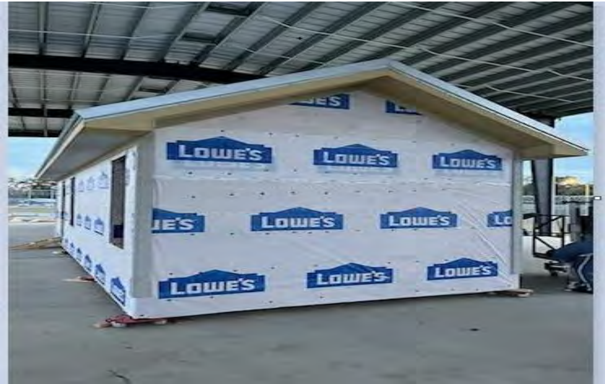
Micro-house with insulation board applied.
