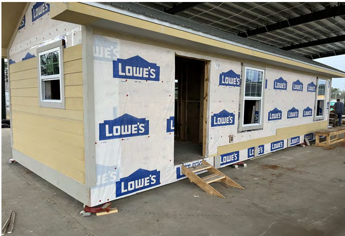
House with exterior siding partially installed.
