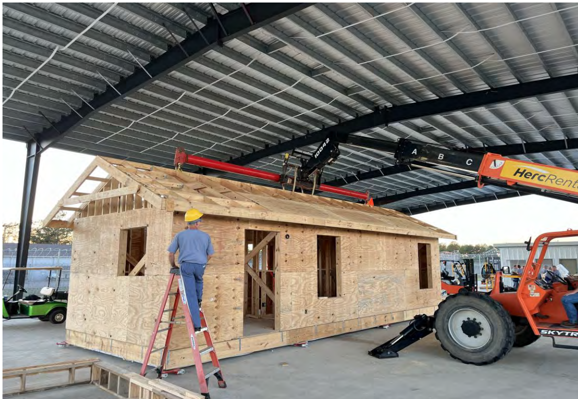
Roof placement on a framed house
